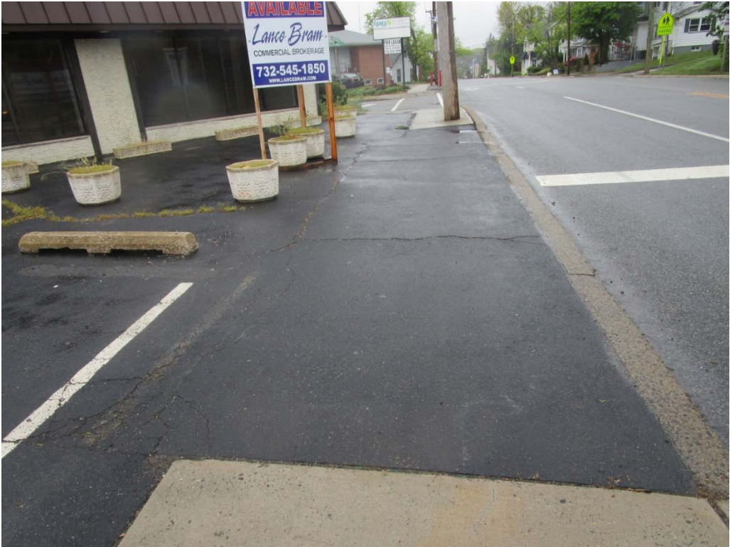
Figure 21 - Wide driveway, Rt. 27 at 11th Ave.
