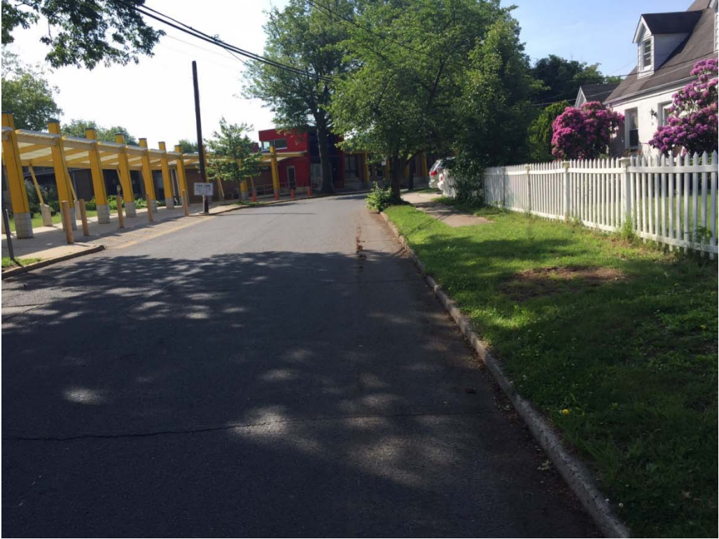
Figure 8 - Missing sidewalk at Irving School entrance, S. 11th Ave.
