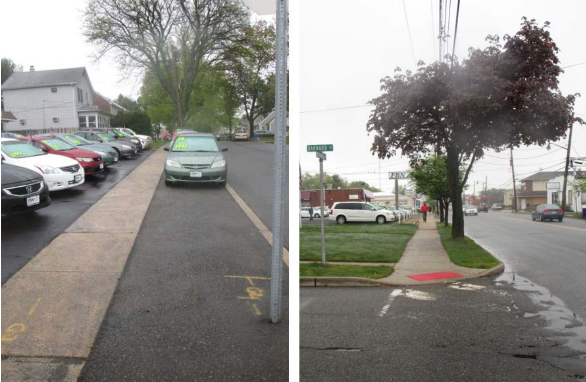
Figure 11 - Unwelcoming and welcoming sidewalks on Woodbridge Ave.
