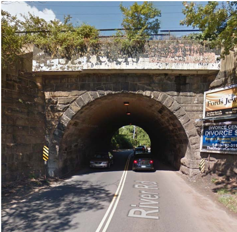
Figure 5 - River Rd. underpass under Amtrak Northeast Corridor rail
